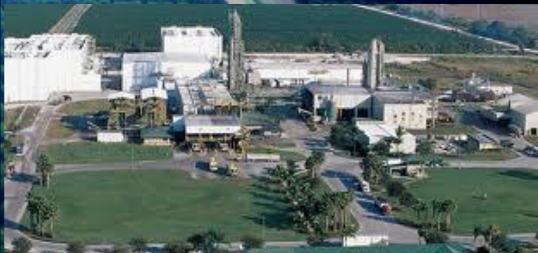
Located in Hendry County, the Southern Gardens processing plant squeezes 650,000 gallons of juice a day.
